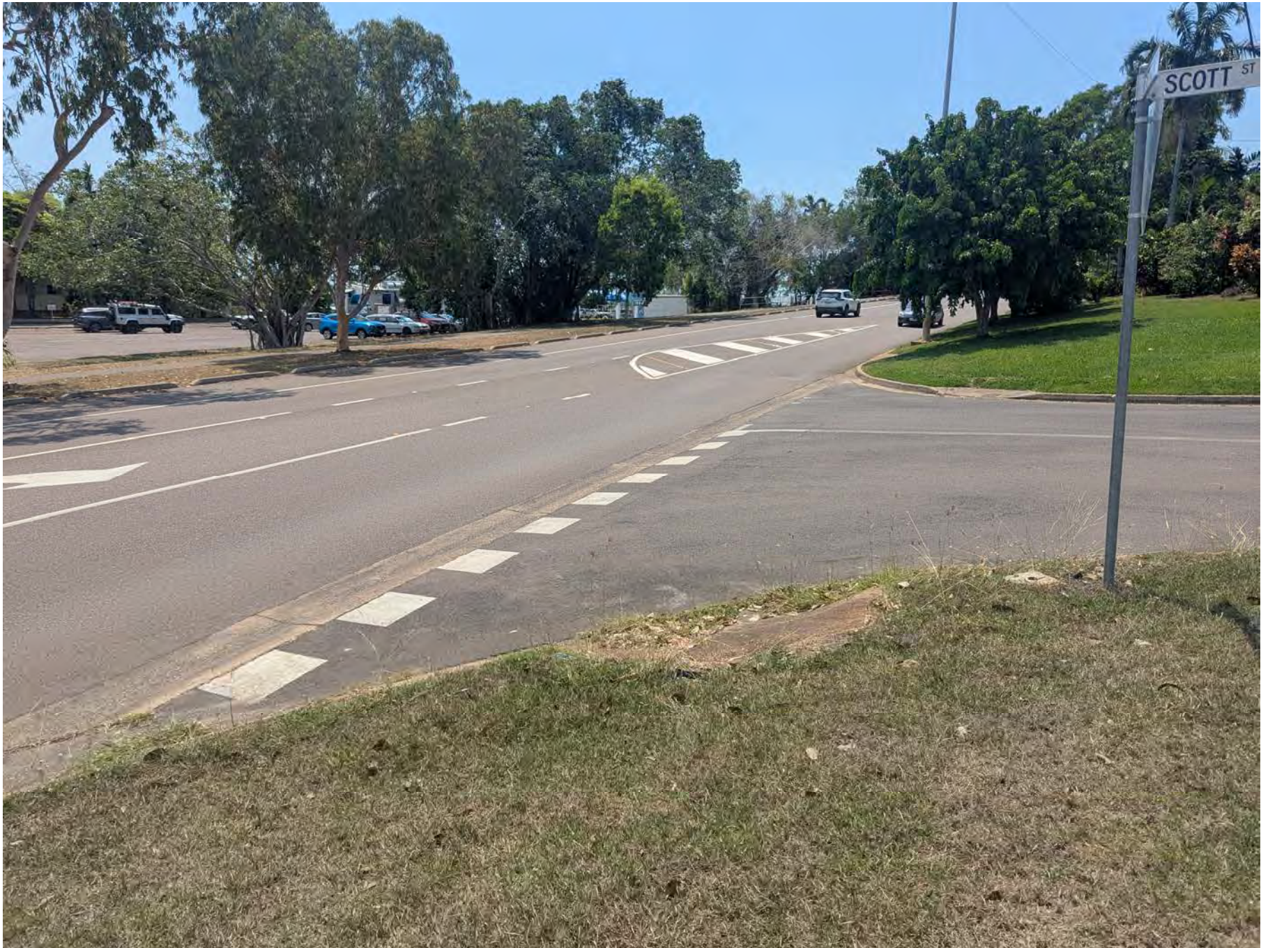
View of East Point Road/Scott Street intersection. Note the pram ramps.
