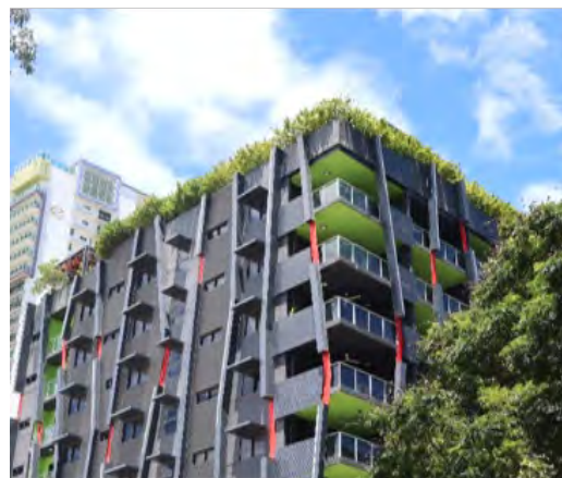
Figure 14: Landscaping of streetscape.
