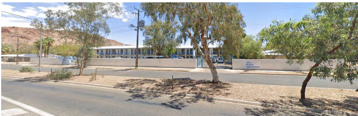
Image 1: Subject site from Gap Road (Source: Google Maps)
