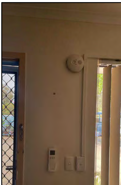
Figure 27 Wall Mounted Smoke Alarm
