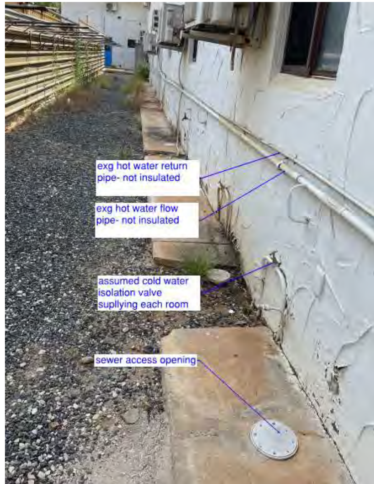
Figure 35 - Back of Building A
