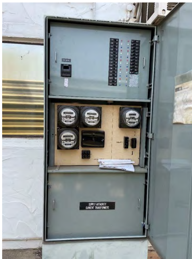
Figure 12 - Main Switchboard
