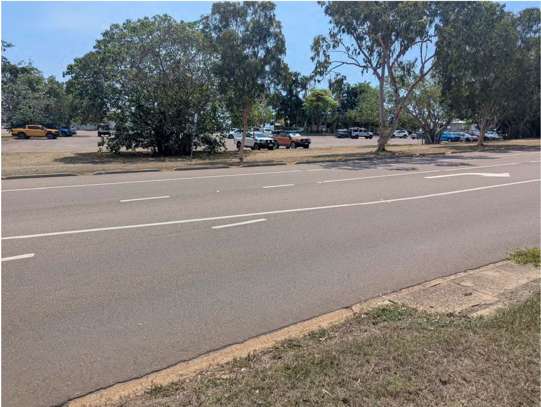
View of East Point Road/Scott Street intersection.
