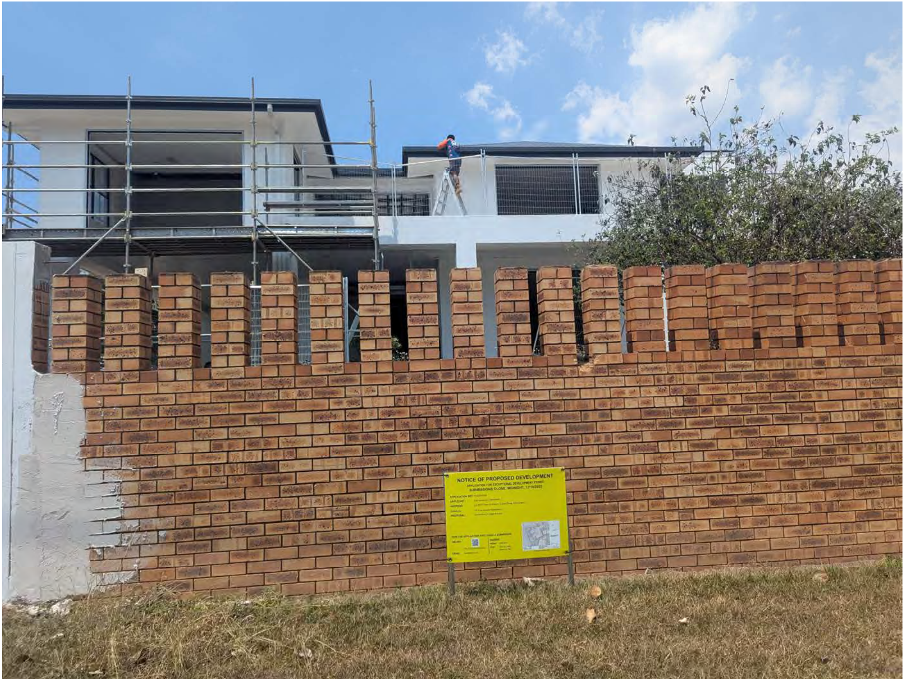
View of East Point Road yellow sign.
