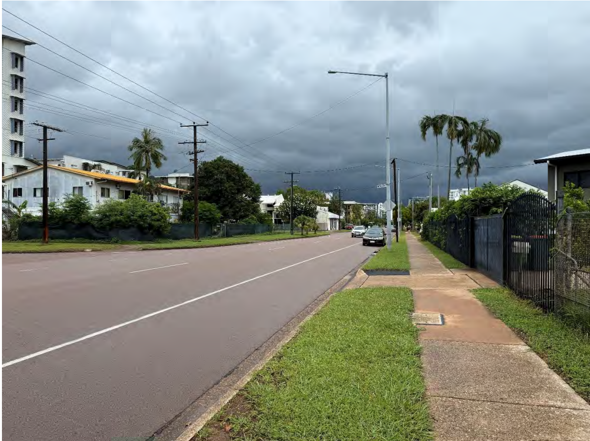
Figure 5 Available Sight Distance (facing Southeast)
